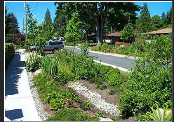
GI for Stormwater Management
